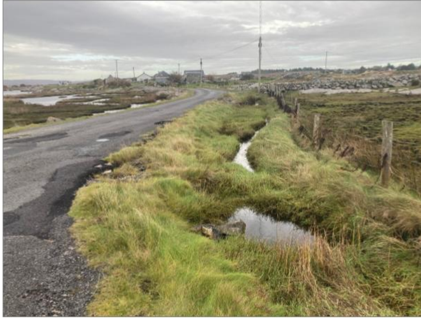
Figure 4.3 View of road drainage ditch (inland verge)
